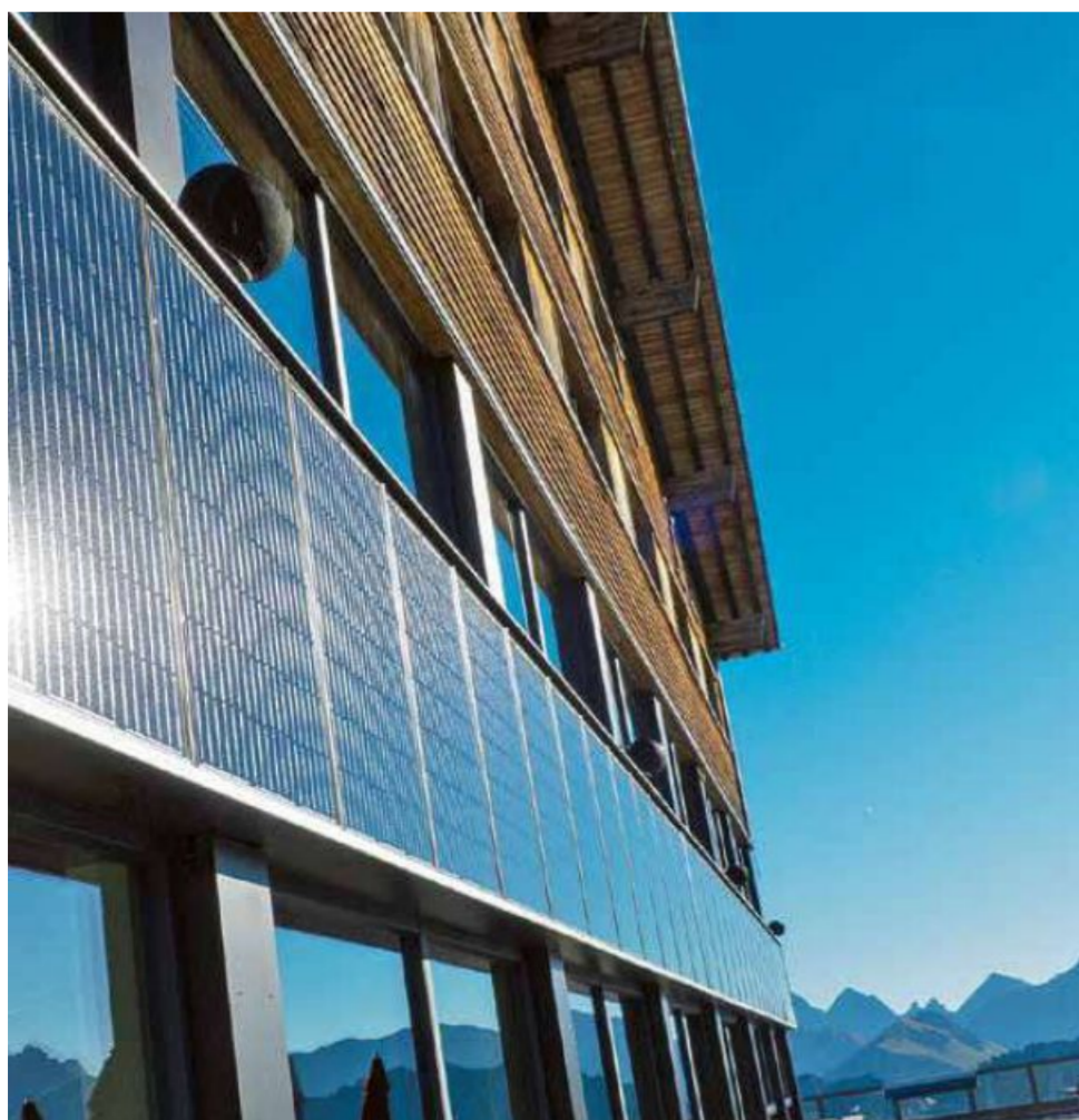
Photovoltaik-Anlage am Fellhorn
